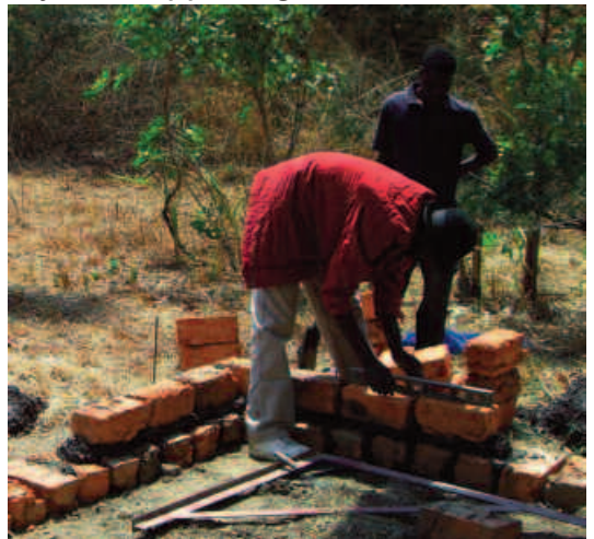
Laying bricks for school in Poleni village.
